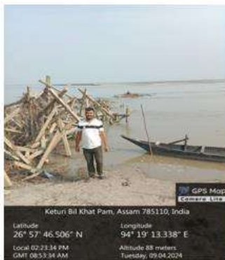
Fig -8. Erosion Control Structure i.e. Porcopine
