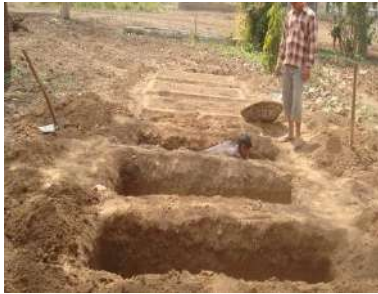
Trenches of 3 m × 1 m × 0.5 m (length, width, depth) size
