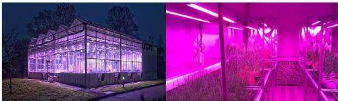
Figure 4. Temperature controlled glasshouses with supplemental lighting consisting of LEDs.
